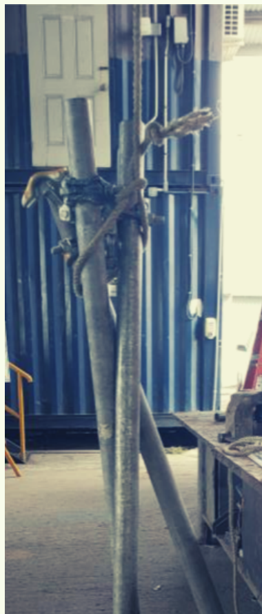
Figure 1: Single lasso tie that was used to lower the pipes.
