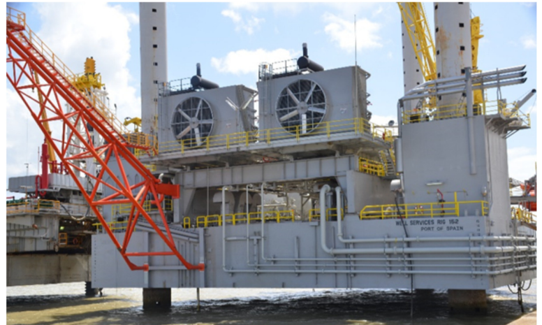
Rig #152 (MOPU) at LABIDCO's Quay Wall.
