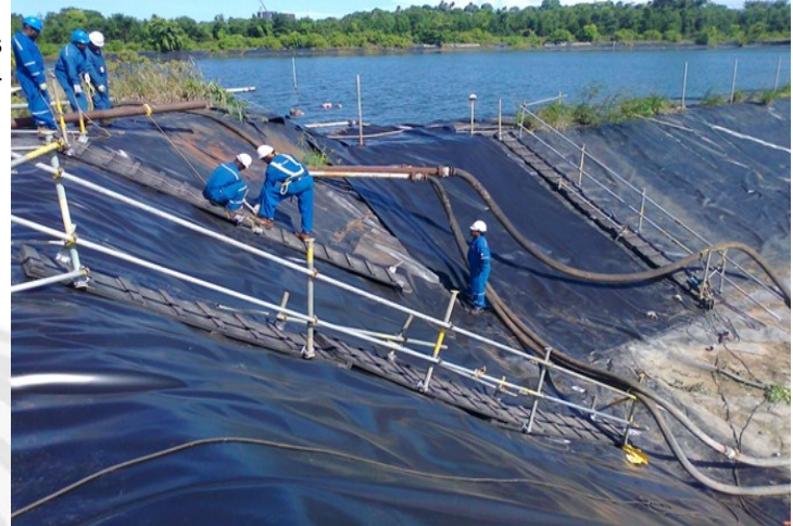
Depicts repair / restoration of Alternative Water Supply Lagoons at Atlantic LNG
